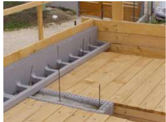
support of the ring beam blocks
