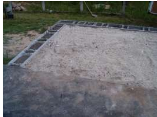
gravel bedding of receptor
