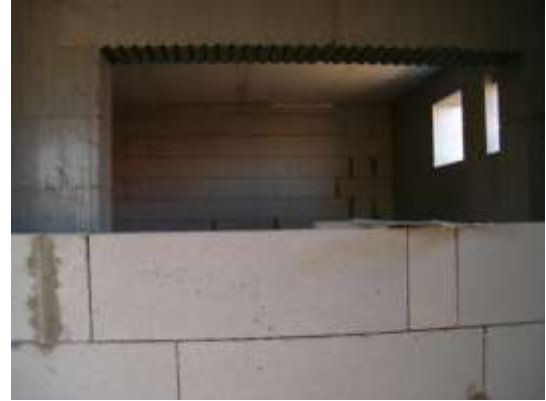
division wall opening
