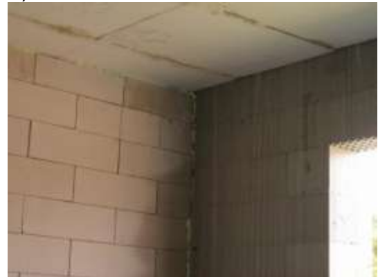
fixing of the division wall
