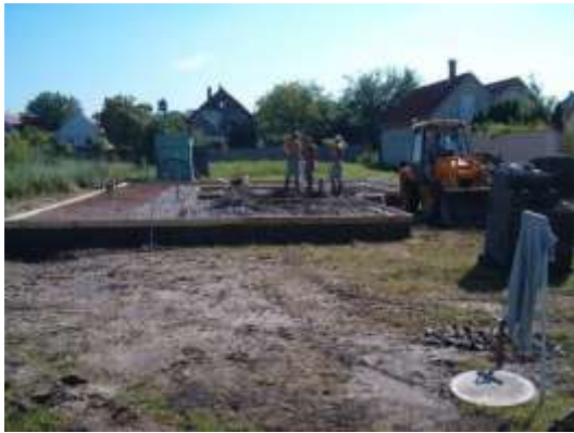
concrete placing
