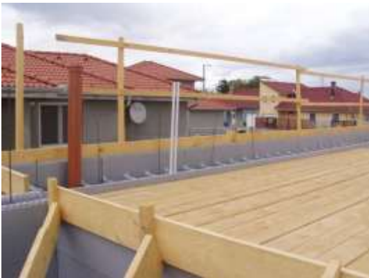
support of the ring beam blocks
